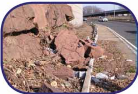
I-280, Garden State Parkway ramp
