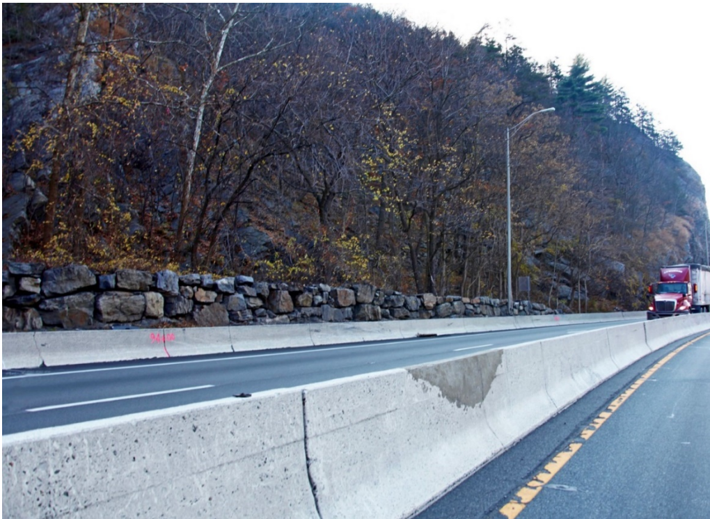
Photograph 2: Area B, looking southeast.
