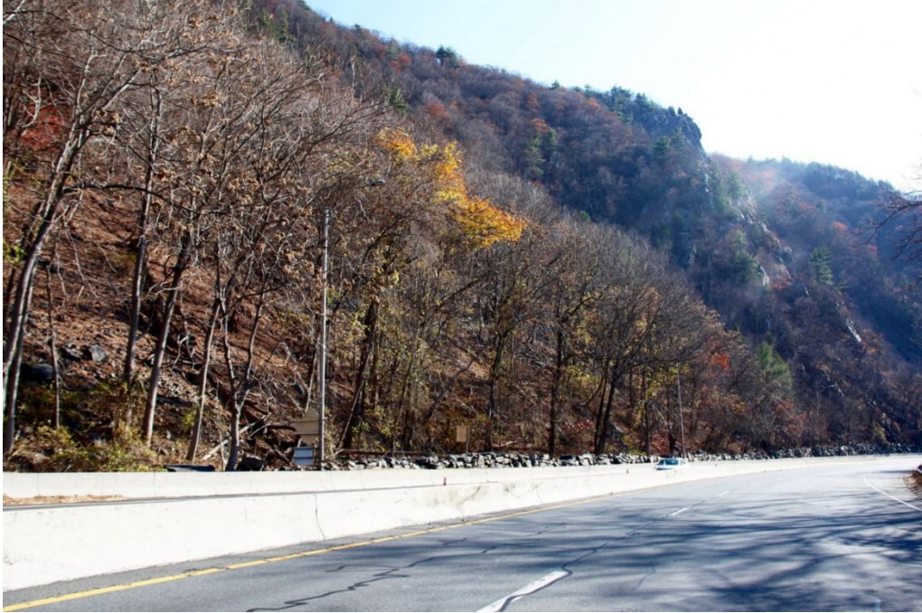
Photograph 1: Area A, looking southeast.
