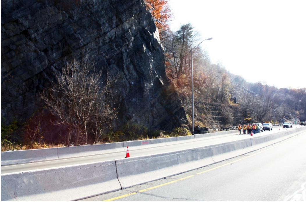
Photograph 3: Areas C and D, looking southeast (note existing gabion wall).
