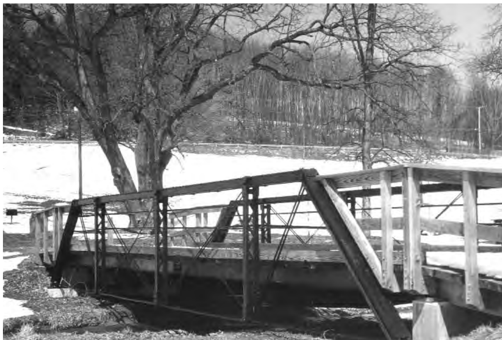
The Augusta Hill Road Bridge at its new location at the Sussex County Fairgrounds, now fulfilling its primary role as a walkway across a slow-moving stream. Wood frame railings have been added at either end to facilitate a decidedly more pedestrian function [Source: New Jersey Department of Transportation].
