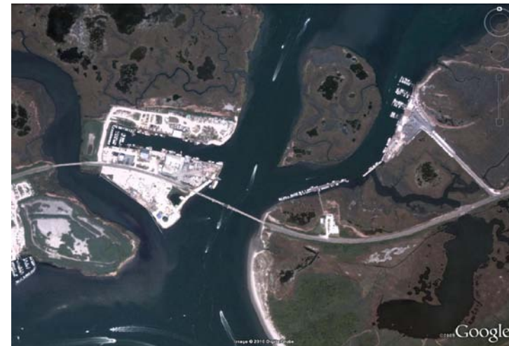
Middle Thorofare Bridge Constrains Commercial Fishing Operations
