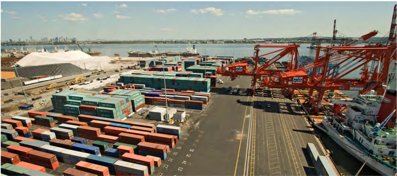
Port Newark Container Terminal, Newark (Source: © David Sailors)
