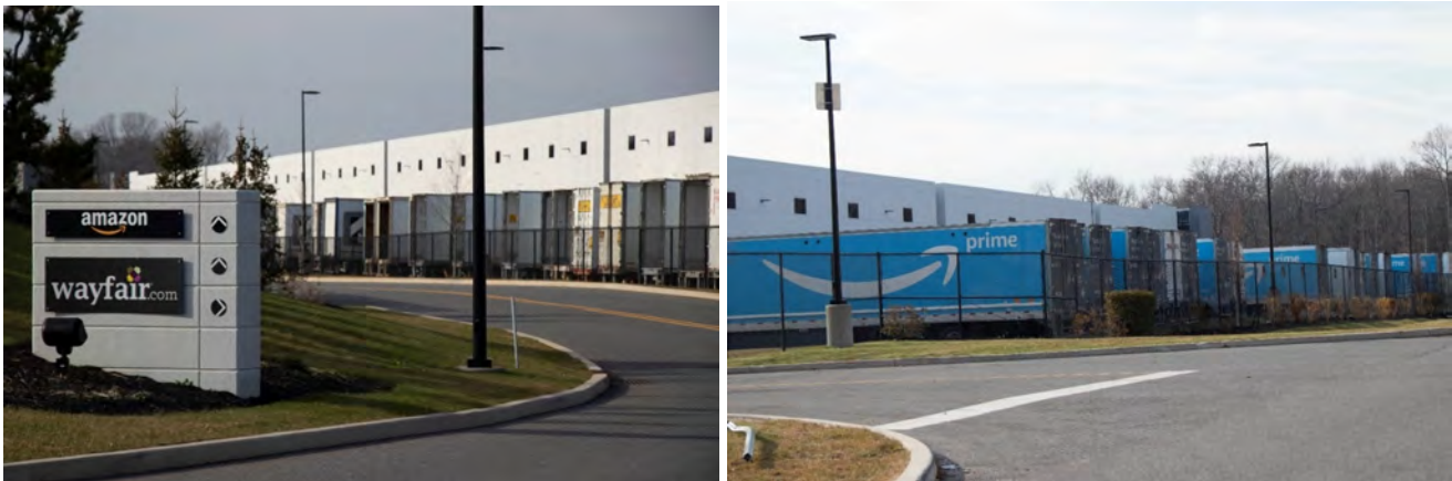
Warehouses and Distribution Centers in Middlesex County, NJ (Source: WSP)
