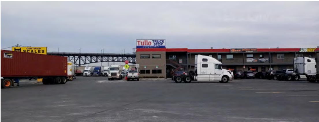
Tullo Truck Stop, Kearny, Hudson County (Source: WSP)
