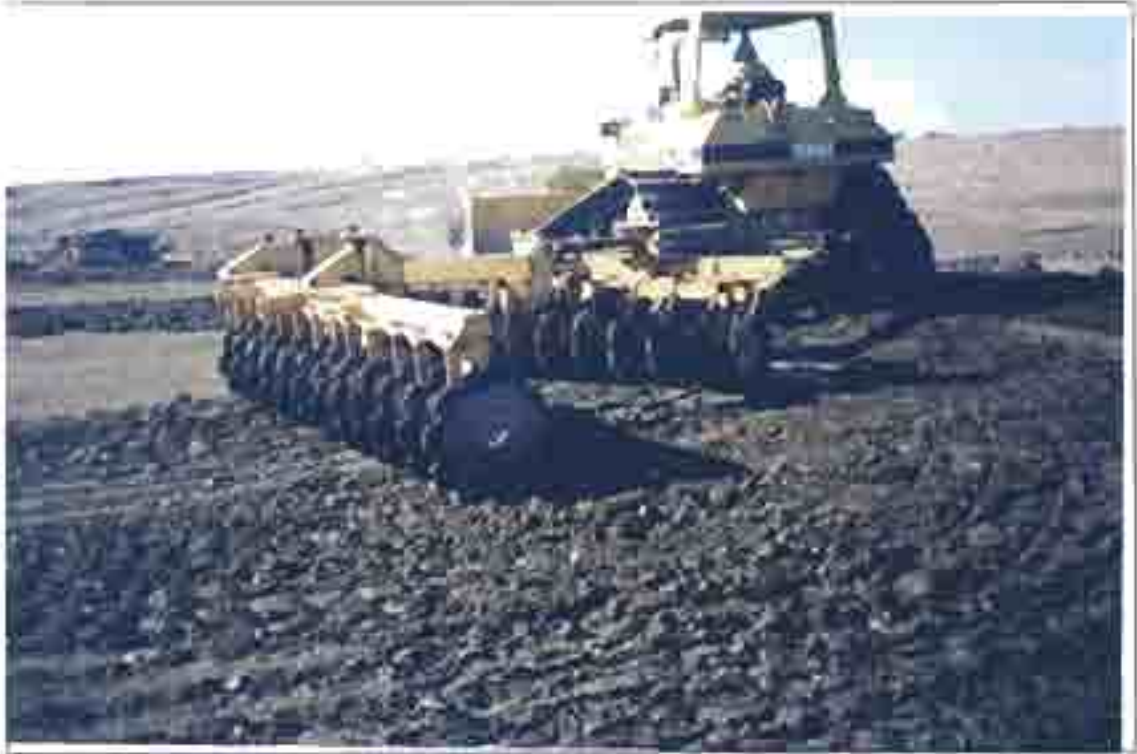
Disking in progress
