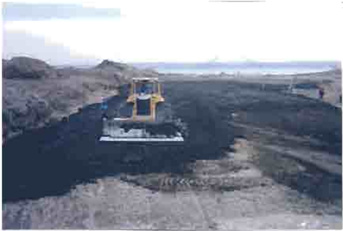
Construction of lift at el. 13.0 ft.
