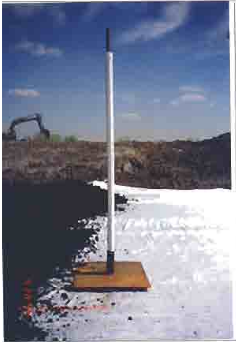
Construction of Piezometer at Location of 5.5 ft Embankment
