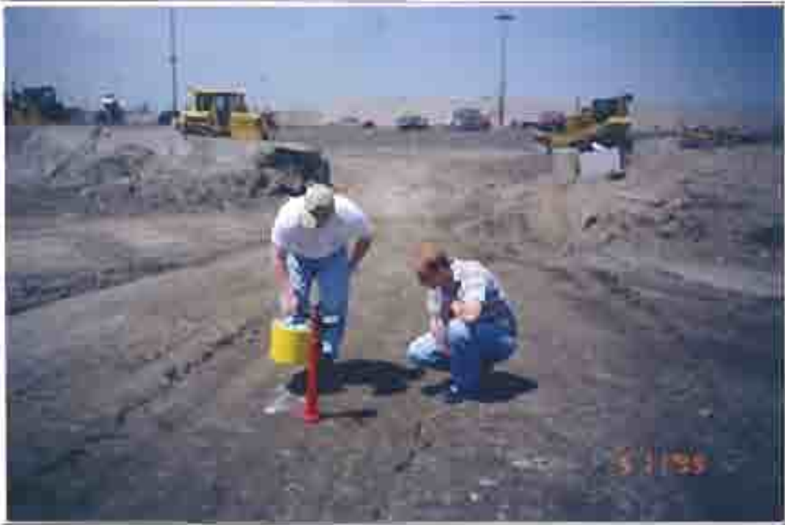
Stiffness Test in Progress (By Rutgers University)
