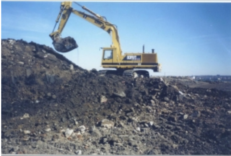
Stockpiling the material available for Embankment construction
