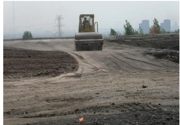
Compaction of PDM grading layer
