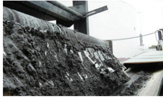
Belt filter press dewatering
