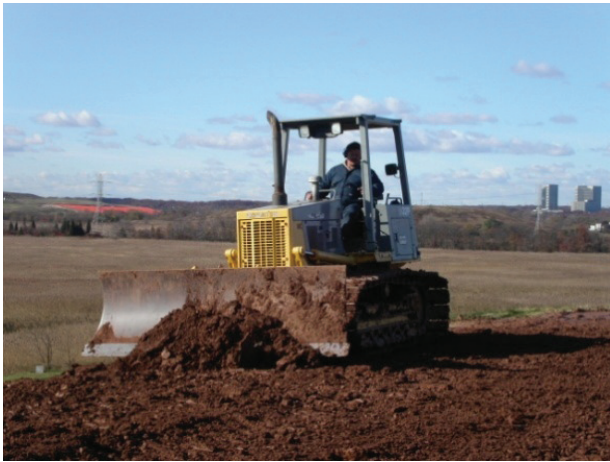
Placing clay on landfill
