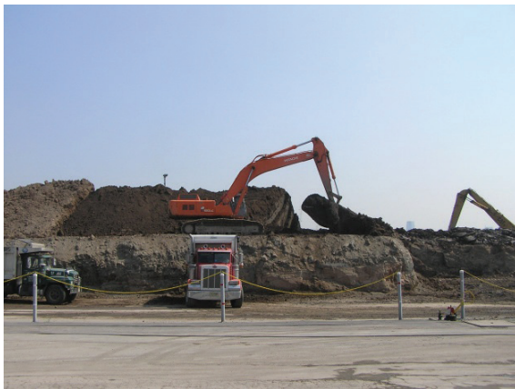
PDM curing operation
