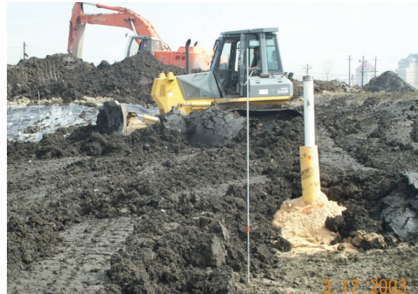
Placing PDM layer at a landfill
