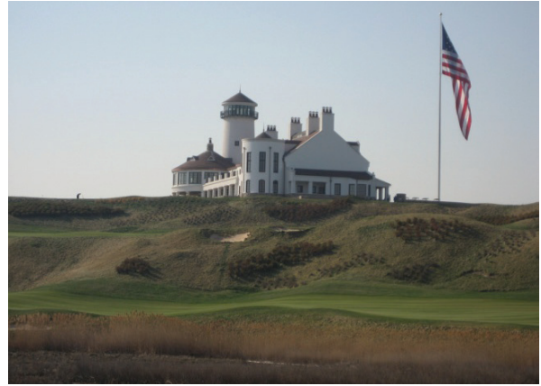
Completed site redevelopment
