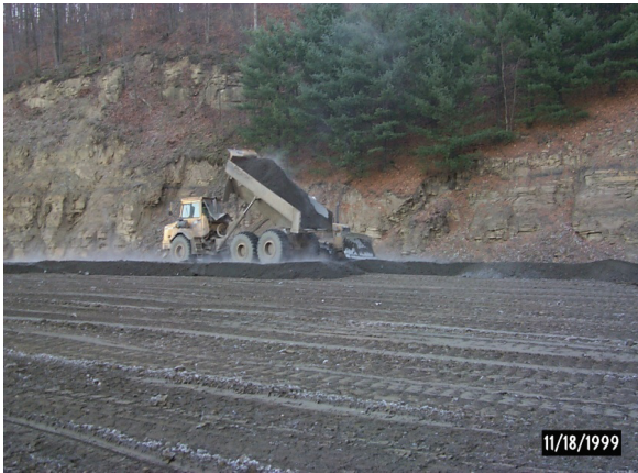
Placing cured PDM in lifts
