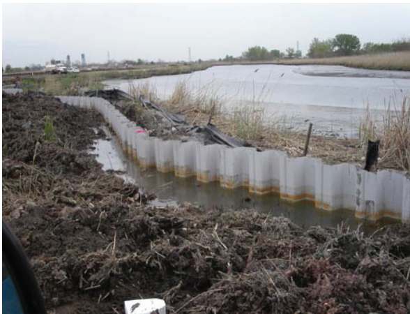
Slurry wall installation
