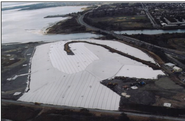
Geotextile membrane on landfill
