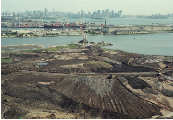
Bayonne site during remediation
