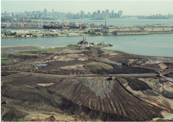
Brownfield remediation with PDM
