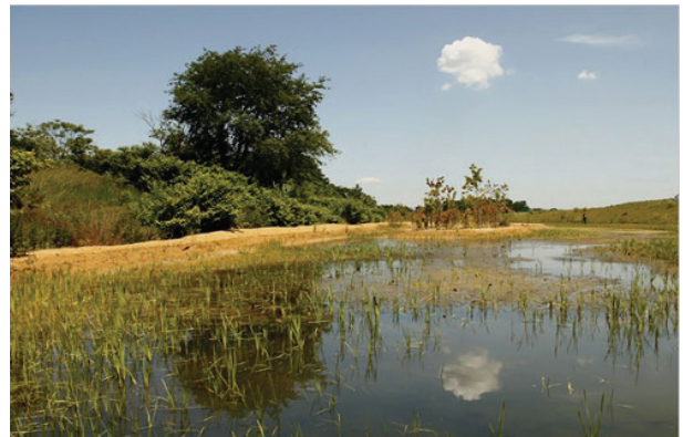
Completed landfill remediation
