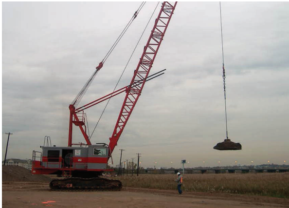
Dynamic compaction of waste
