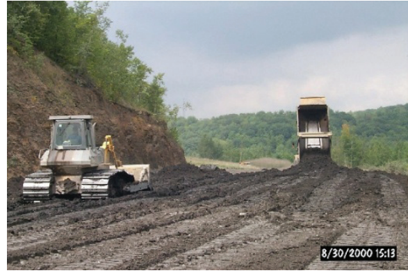
Placing PDM on the highwall
