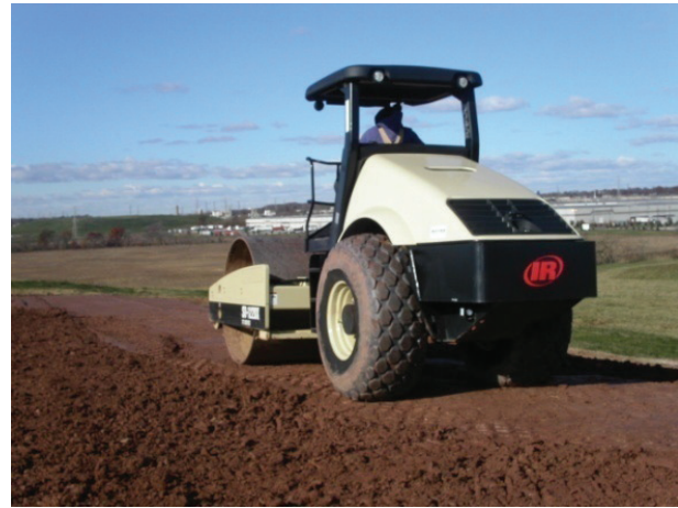
Compacting clay cap
