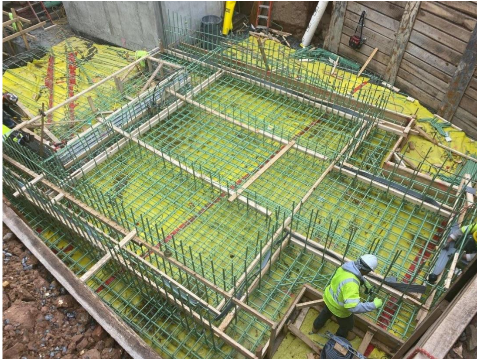
Figure 2-3: Reinforced Steel installed for Escalator and Staircases foundation slab.
