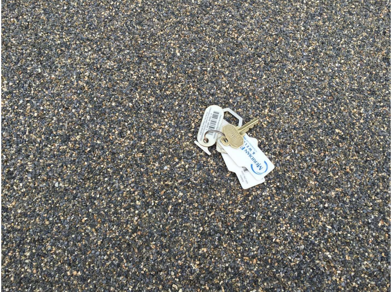
Figure 1 – High Friction Surface Treatment (HFST)
