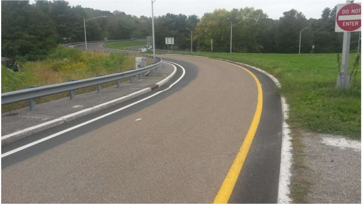
Figure 2 – HFST on Asphalt Surfaced Pavement
