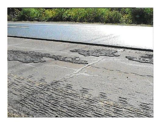
Scabbing occurs when an existing layer of pavement is not fully removed during the milling operation. The RE should discuss scabbing and how to address this issue during the pre-paving meeting so a plan is in place prior to starting the milling operation.
