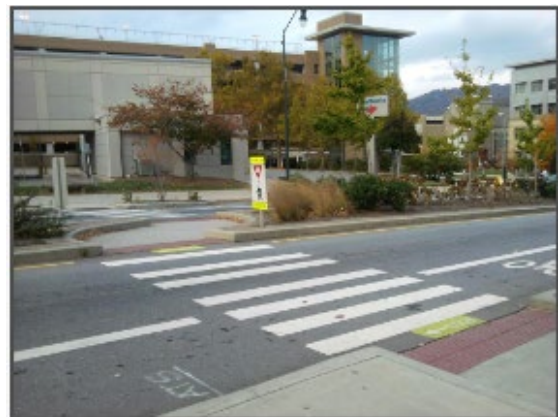
Median refuge island
