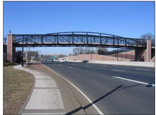
Figure 6-1 - A pedestrian bridge over Route 18 links the community with a riverfront park.
