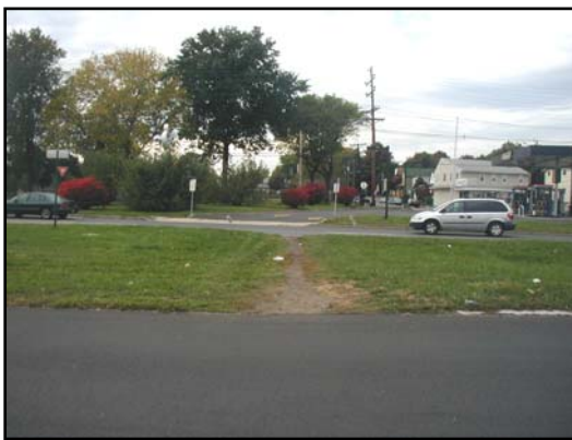
Figure 4-3 - Trampled grass can provide indications of unmet pedestrian needs and possible safety issues to address.
