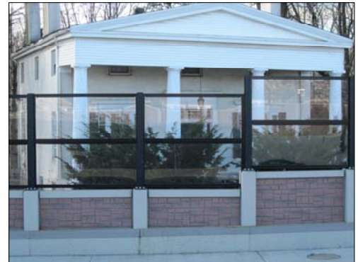
Figure 6-3 - Clear noise walls minimize visual and auditory effects along Route 18 in New Brunswick.
