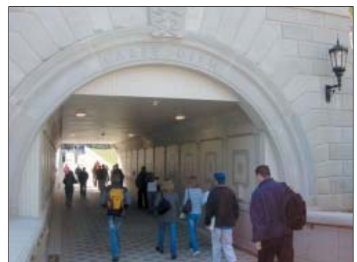
Figure 6-2 The final design for the Route 71 Pedestrian Tunnel at Monmouth University addressed the historic and social contexts of the area.
