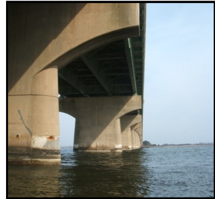
Bay Bridge girders
