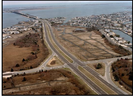
Marsha Drive intersection
