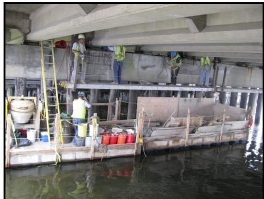
Pier cap repair – trestle bridges
