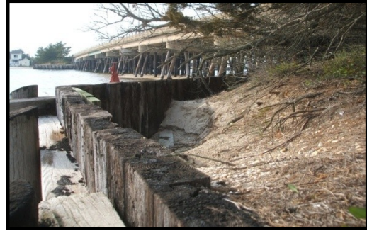
Timber bulkheads
