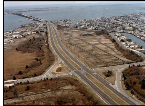
Marsha Drive intersection
