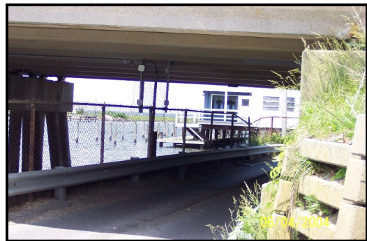
Access road under bridge
