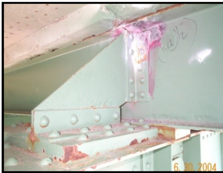
Fatigue cracking
