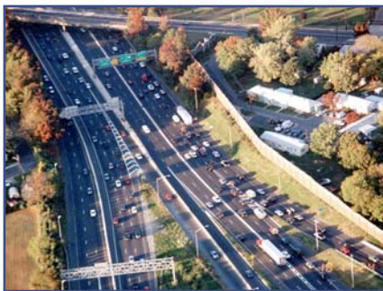
Source: Dewberry, Existing conditions at I-295/I-76/Route 42 Interchange
