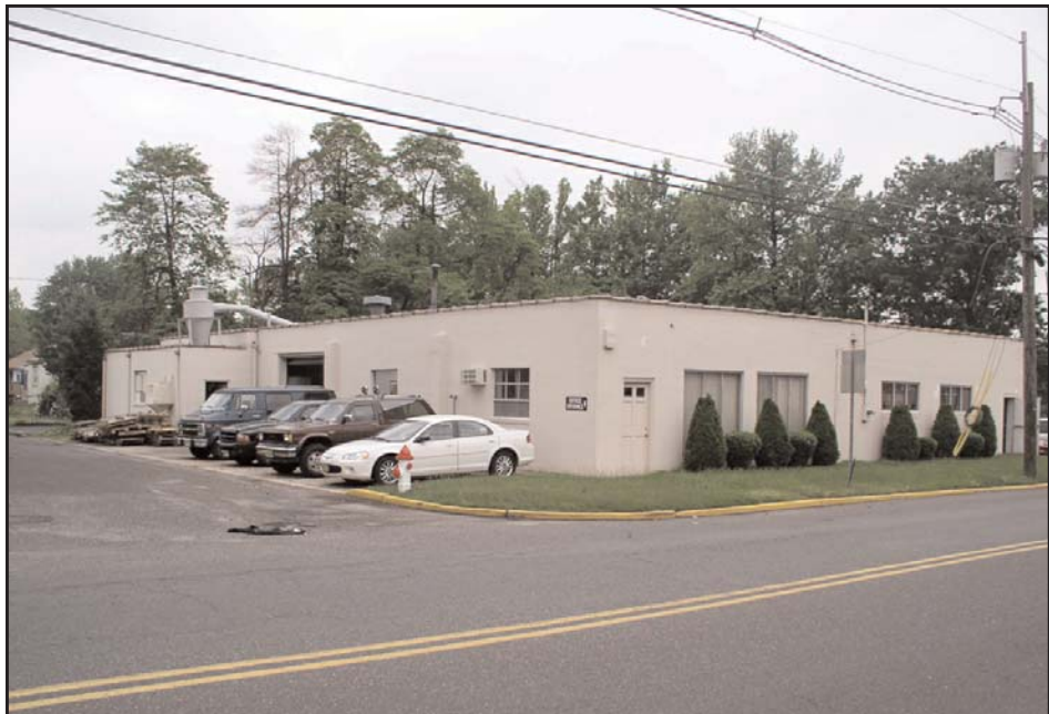
Plate 16: 700 Creek Road. View looking southwest (May 2004).
