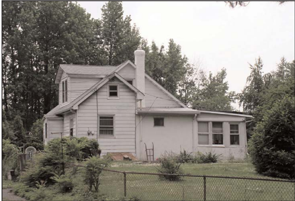
Plate 21: 48 Essex Avenue. View looking south (May 2004).
