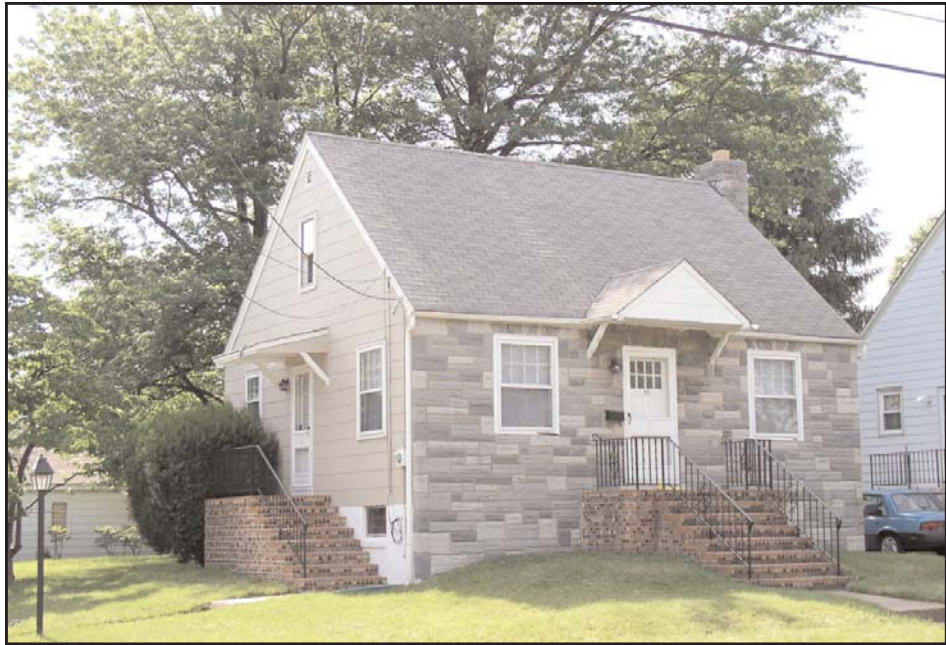
Plate 5: Representative dwelling in the Linwood Tract District II. View looking northwest along Harding Avenue (May 2004).
