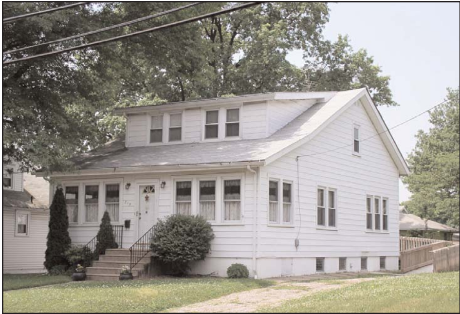
Plate 35: 713 Bell Road. View looking southwest (May 2004).
