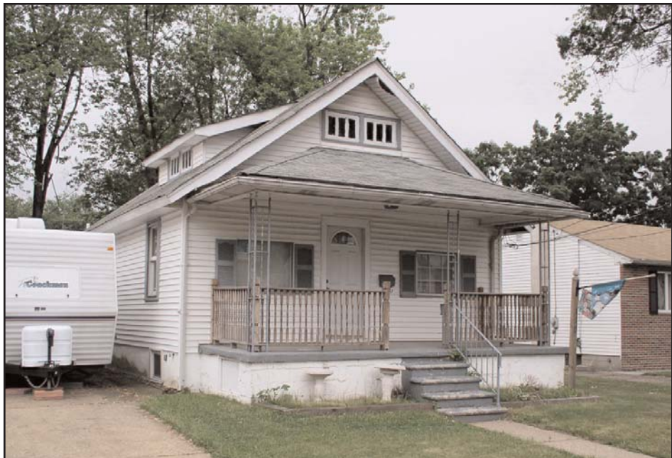
Plate 40: 110 Cleveland Avenue. View looking southeast (May 2004).
