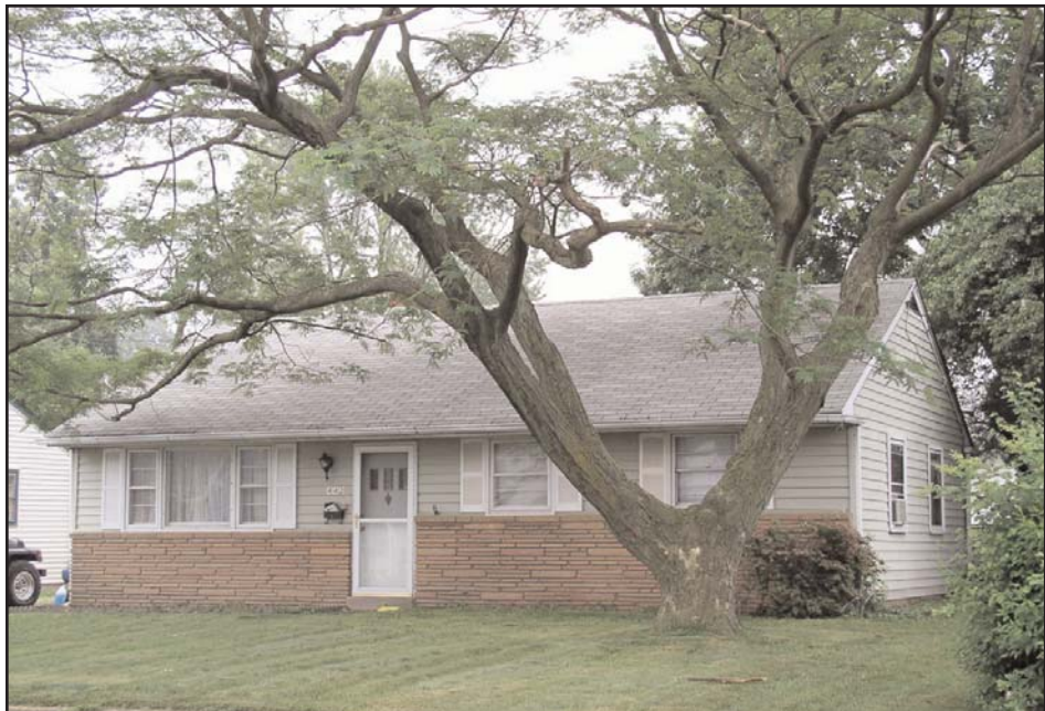
Plate 2: Representative dwelling in the Bellwood Park District. View looking south along Windsor Drive (May 2004).
