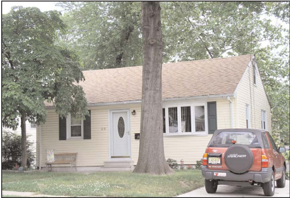
Plate 49: 128 Roosevelt Avenue. View looking northeast (May 2004).
