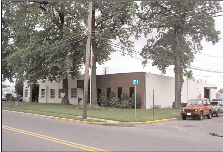
Plate 15: 640 Creek Road. View looking southeast (May 2004).
