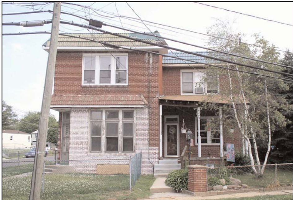
Plate 34: 202-206 Baird Avenue. View looking northeast (May 2004).
