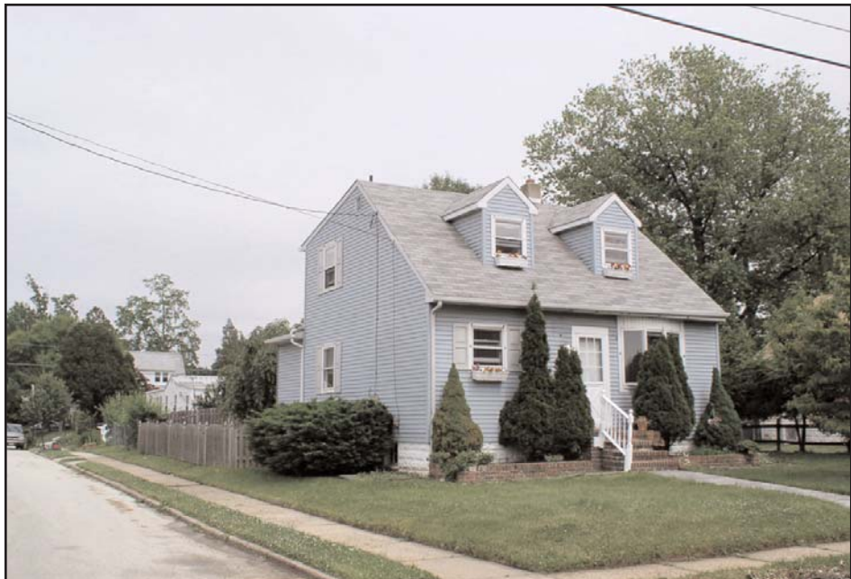
Plate 38: 102 Cleveland Avenue. View looking southeast (May 2004).
