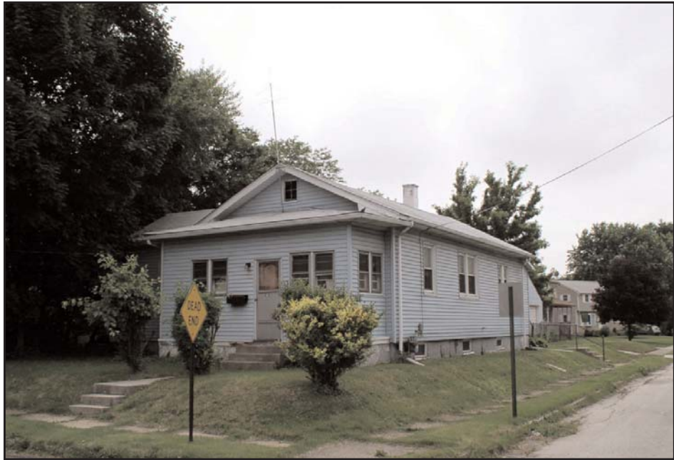
Plate 37: 101 Cleveland Avenue. View looking southwest (May 2004).
