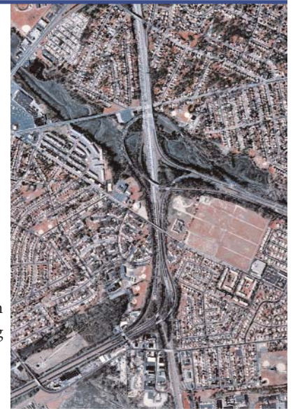
Source: NJDEP Bureau of Geographic Information and Analysis, Current aerial of I-295/I-76/Route 42 Interchange
