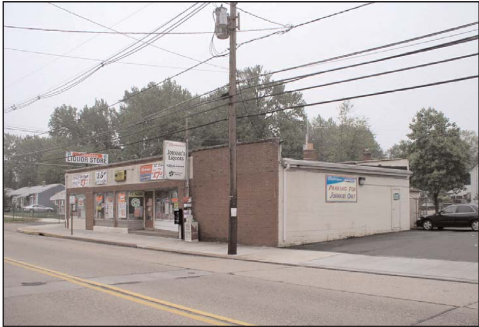
Plate 31: 834 West Browning Road. View looking southeast (May 2004).
