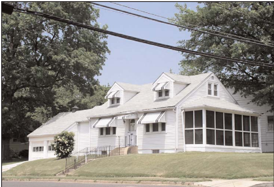
Plate 36: 715 Bell Road. View looking northwest (May 2004).
