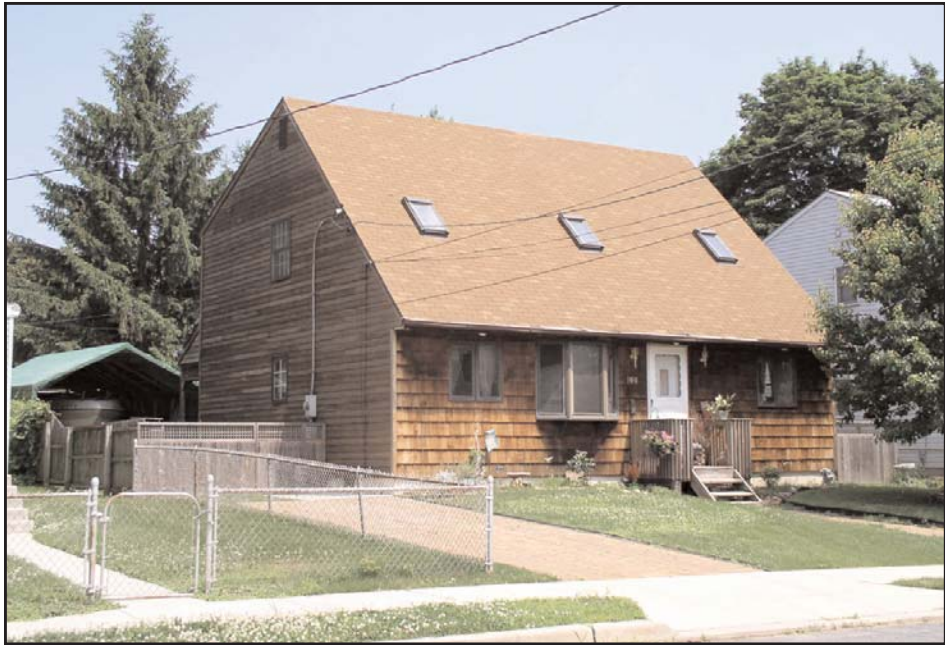
Plate 45: 106 Harding Avenue. View looking southeast (May 2004).
