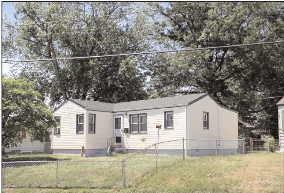
Plate 4: Representative dwelling in the Linwood Tract District I. View looking northeast along Winthrop Avenue (May 2004).
