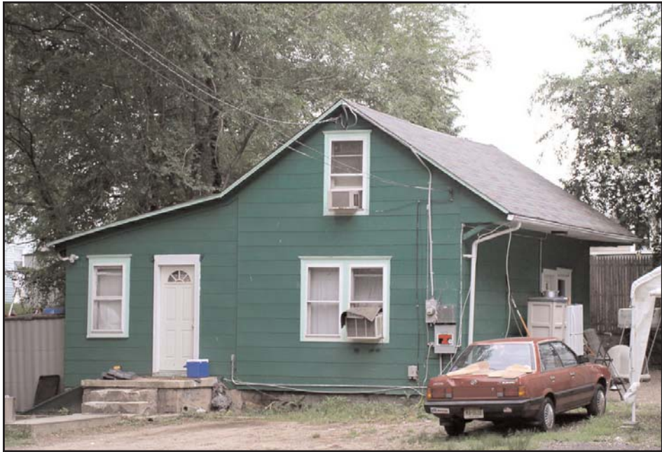
Plate 41: 328 Emerson Avenue. View looking northwest (May 2004).
