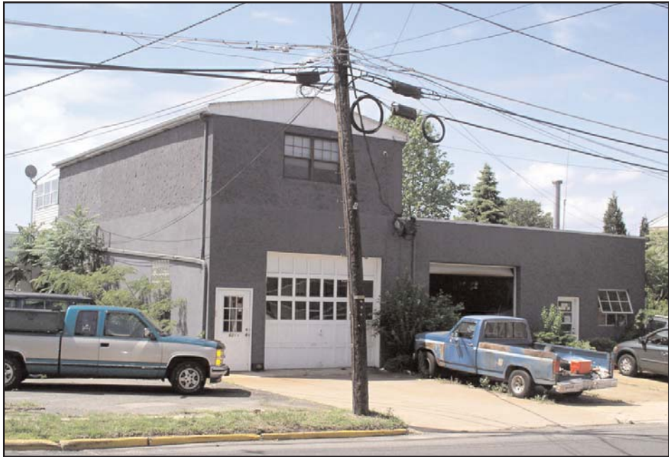
Plate 13: 620 Creek Road. View looking southwest (May 2004).
