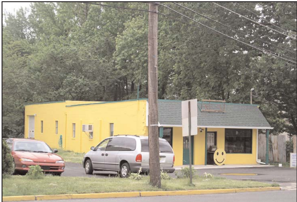
Plate 18: 708 Creek Road. View looking southwest (May 2004).
