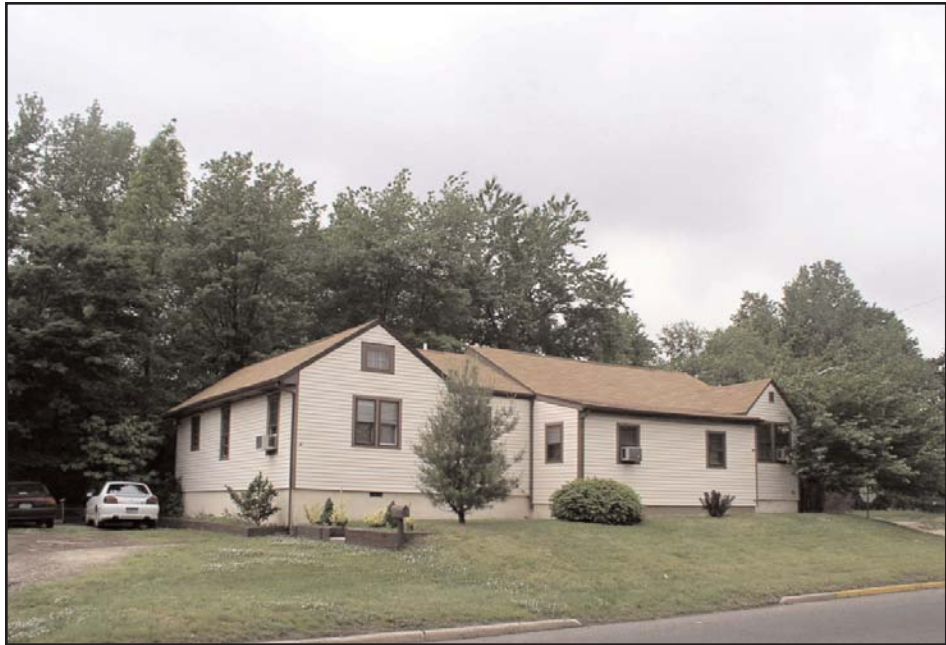
Plate 17: 701 Creek Road. View looking north (May 2004).
