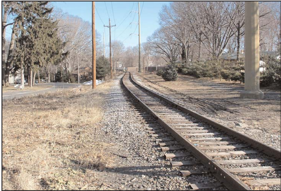
Plate 9: Camden County Railroad. View looking north from Anderson Avenue (September 2003).
