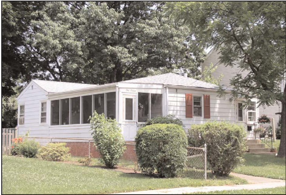
Plate 47: 116 Harding Avenue. View looking southeast (May 2004).
