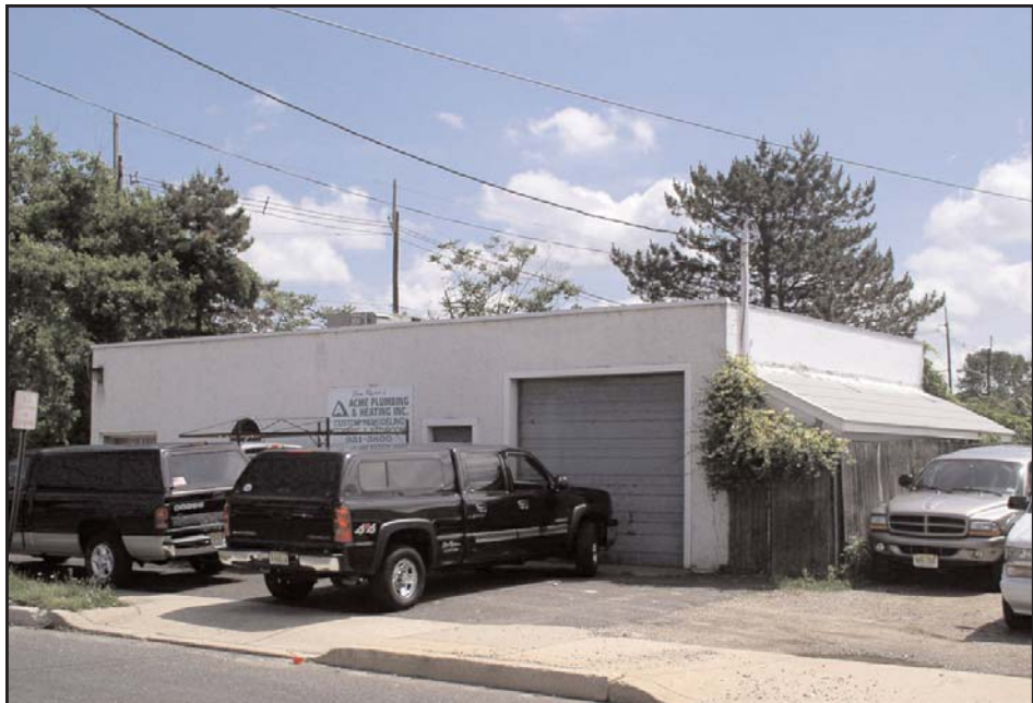
Plate 12: 612 Creek Road. View looking northeast (May 2004).
