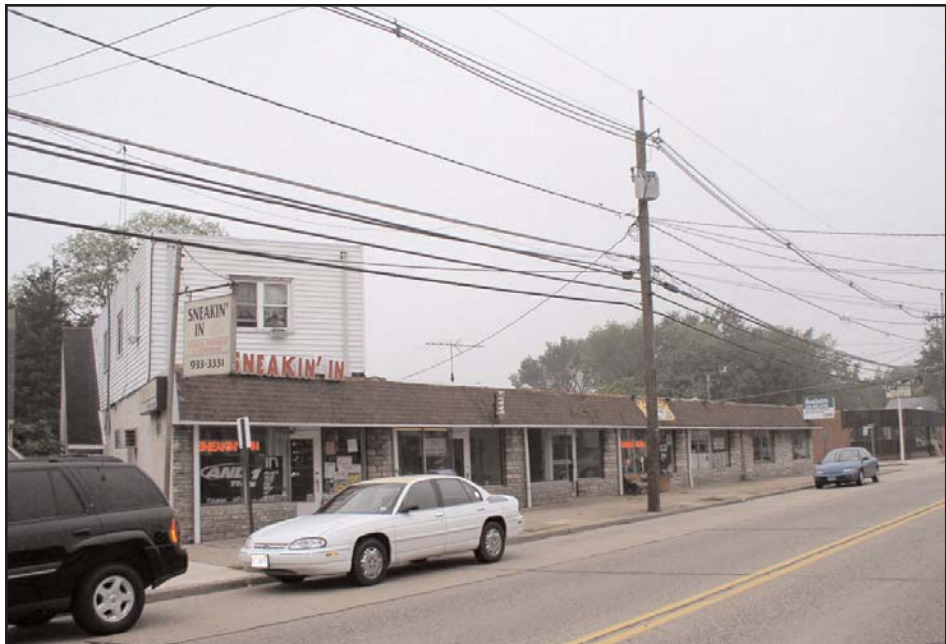
Plate 32: 846-856 West Browning Road. View looking southwest (May 2004).
