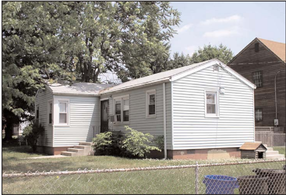
Plate 43: 102 Harding Avenue. View looking southeast (May 2004).
