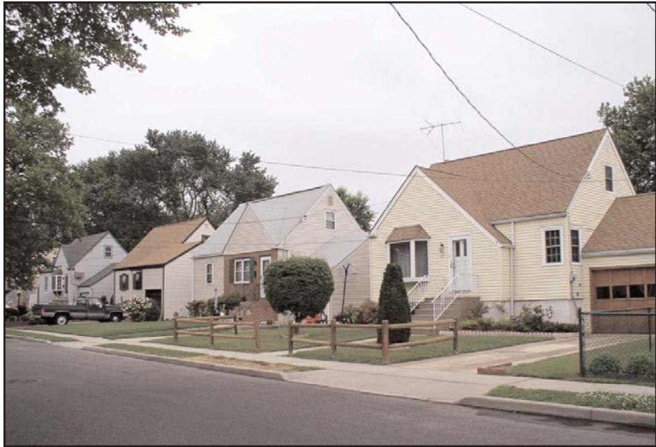
Plate 3: Streetscape along Union Avenue in the Crescent Park District. View looking east (May 2004)
