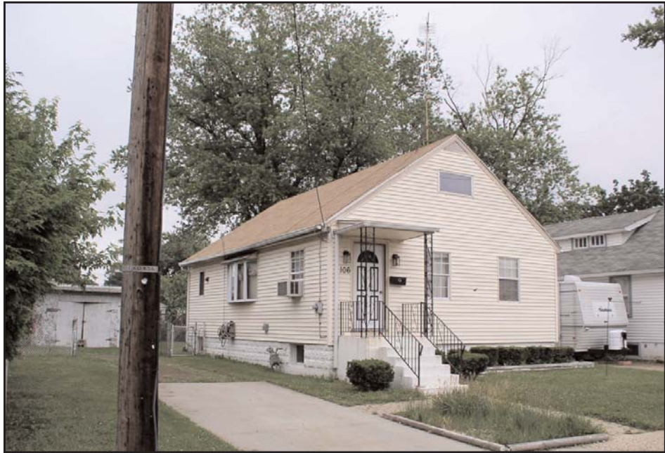
Plate 39: 106 Cleveland Avenue. View looking southeast (May 2004).
