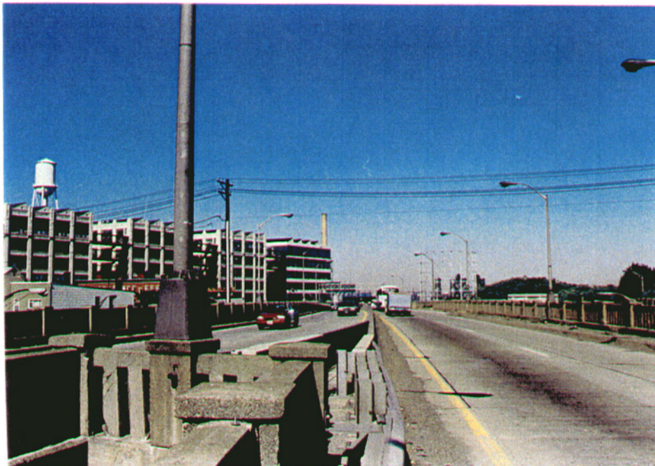
a) Typical roadway and railing configuration on low-level viaduct of Pulaski Skyway in Jersey City.
