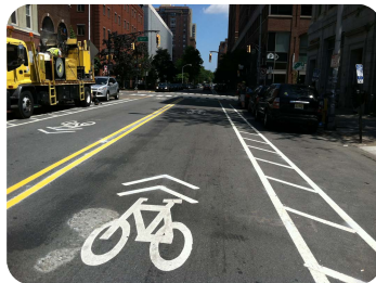
Shared Lane Markings in Hoboken, NJ Image: The RBA Group
