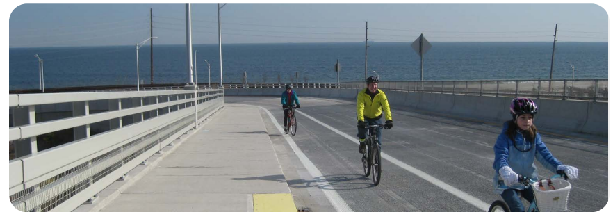
Image: Route 36 Bridge, The RBA Group
