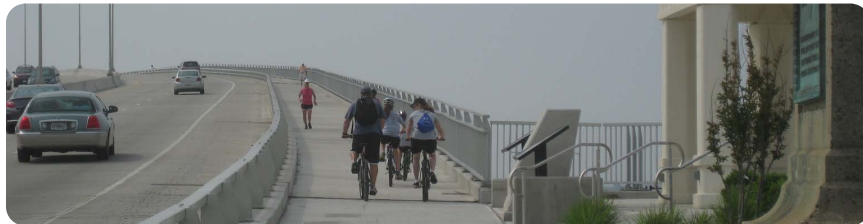
Image: Route 52 Bridge, The RBA Group
