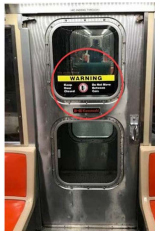
Figure 2-5: Enhanced SEPTA door warning following this accident
