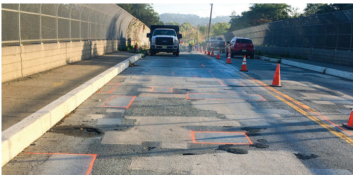
Pictured: Crews marking areas of delaminated concrete as part of Bridge Preventive maintenance on North Gaston Ave over I-287 in Bridgewater, Somerset County.
