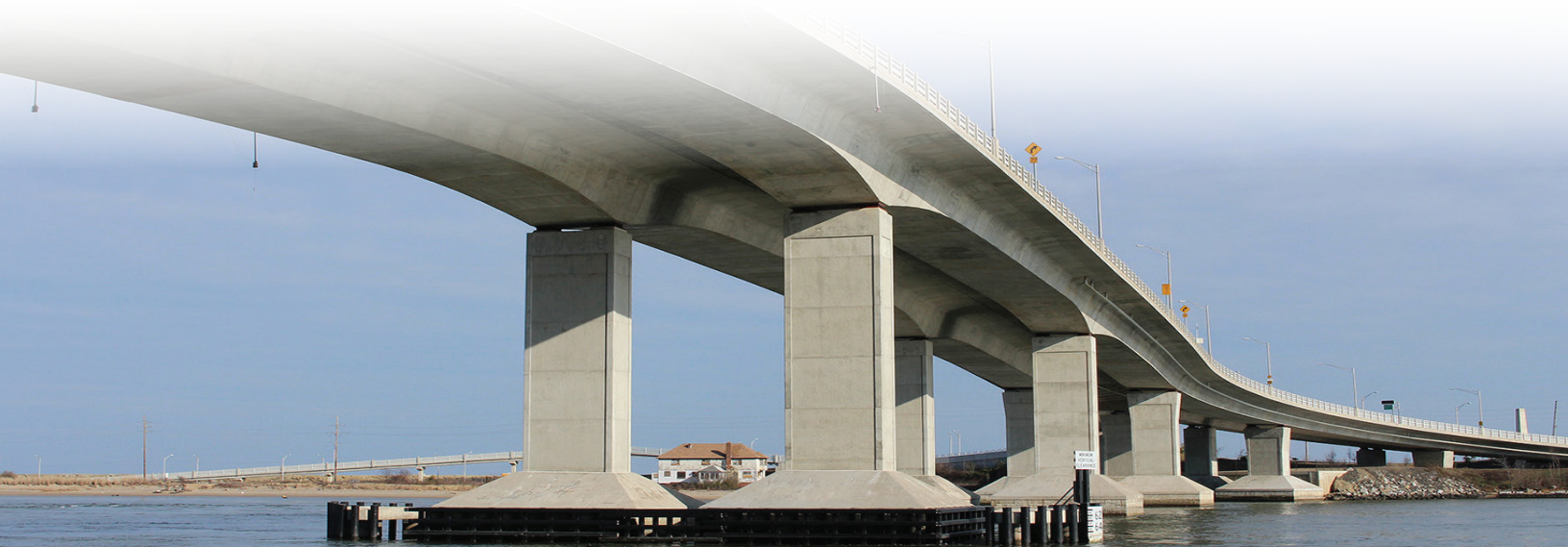
Pictured: Route 36 Highlands Bridge in Monmouth County.
