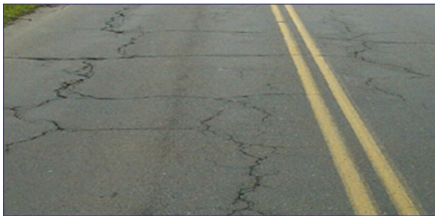
Cracking
